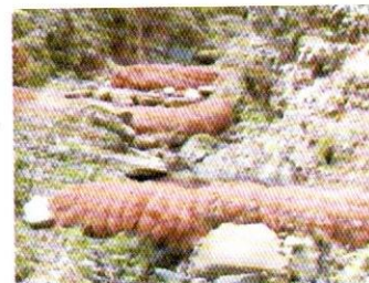
(Pirul check dam)
